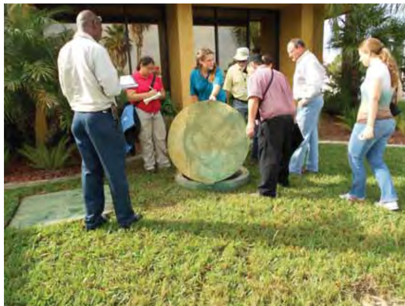
WTW Team inspecting lift station.
