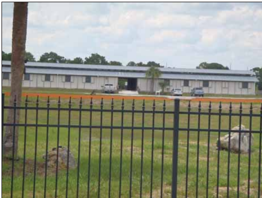
Figure 88. Crestwood Stables Barn.
