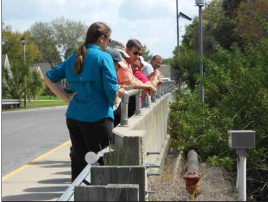
Figure 29. WTW Team at Park Forest Bridge. Air-Release Valve.
