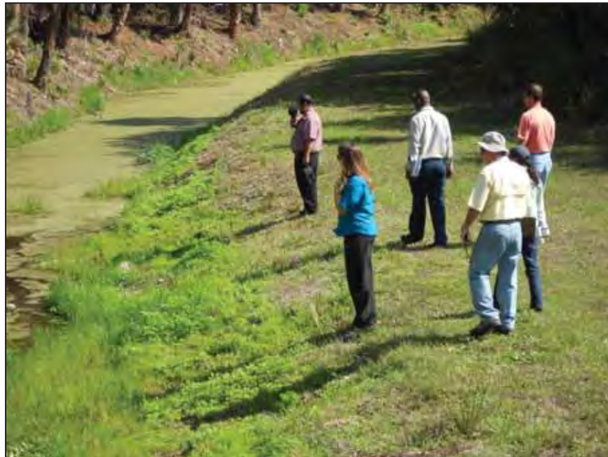
Figure 12. WTW Team Inspecting Englewood Lateral.
