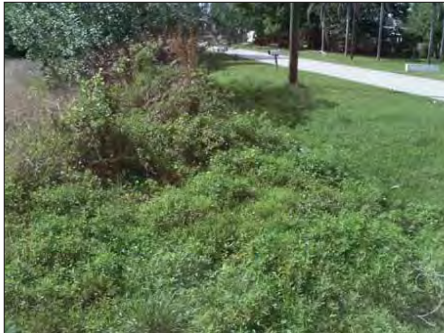
Figure 21. Drainage Ditch South of E. Riverview Ave. and West of Liberty St.
