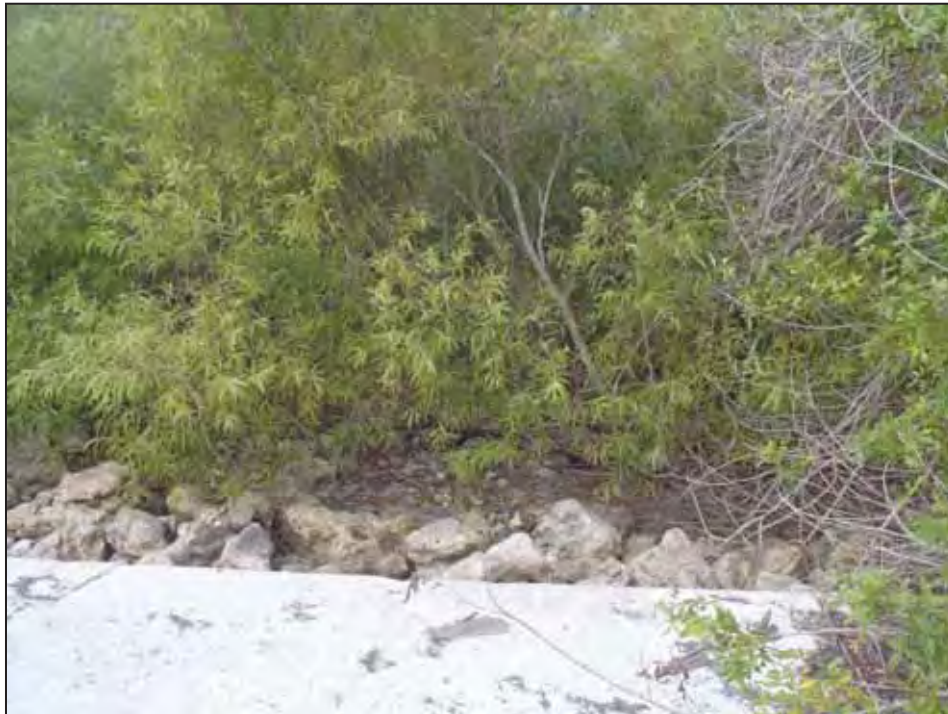
Figure 64. Englewood Lateral at Confluence with Gottfried Creek-Below Weir.
