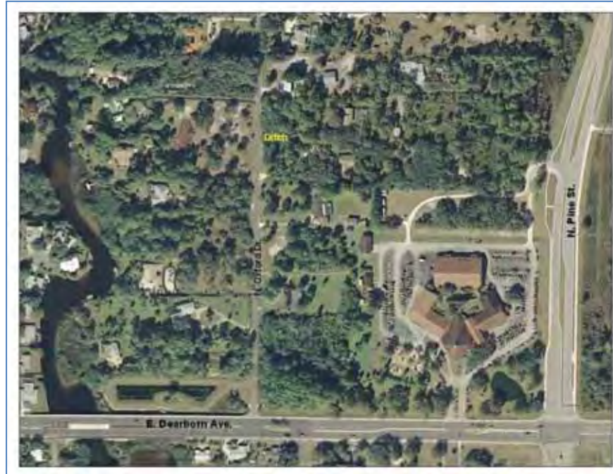
Figure 51. North Oxford Stormwater Ditch-Aerial View.
