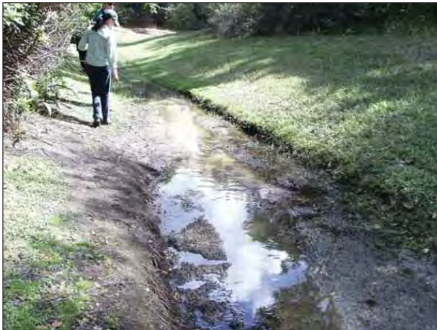
Figure 18. Foxwood Stormwater Ditch – View Toward Downstream.
