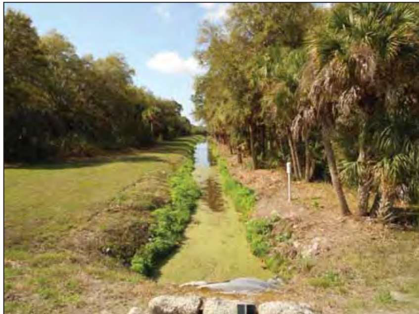
Figure 10. Englewood Lateral at Tangerine Woods Boulevard – Upstream.
