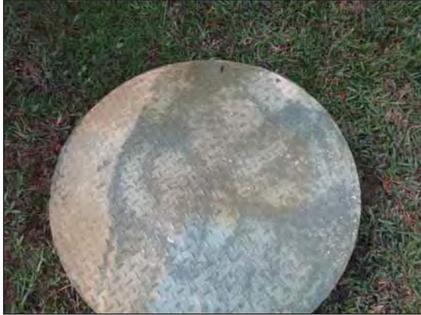
Figure 3. Private Lift Station – Provision Eye Center
