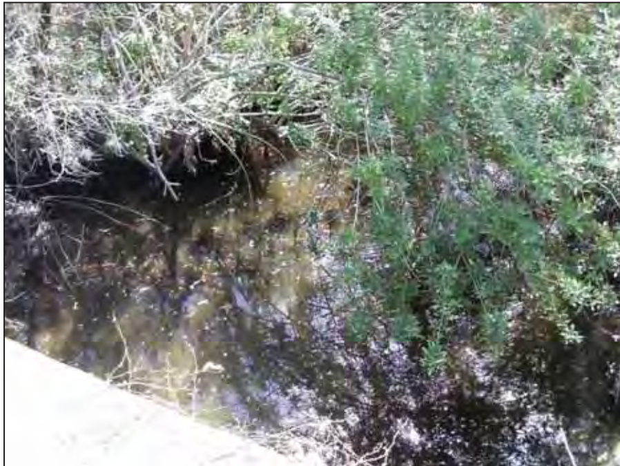
Figure 32. Gottfried Creek at Park Forest Bridge.
