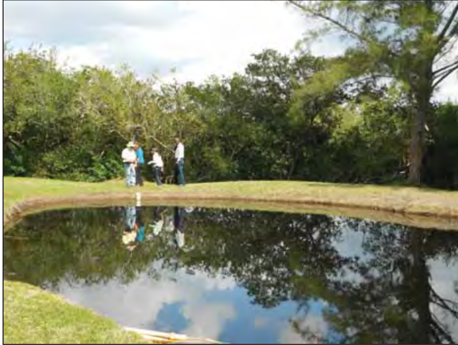
WTW Team Inspecting Berm Around Pond.
