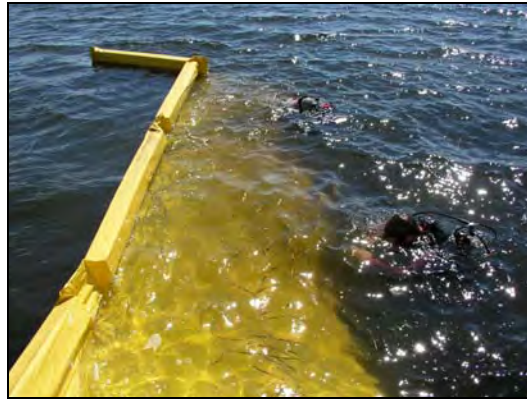
Fig 3. Containment boom showing surface floatation and side panel
