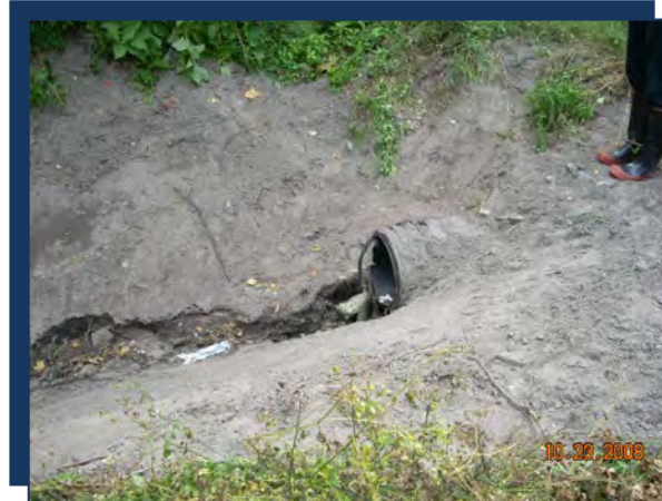
Photo: AC09 Culvert Outfall
