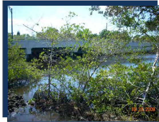
Photo: GC02 Downstream Culvert
