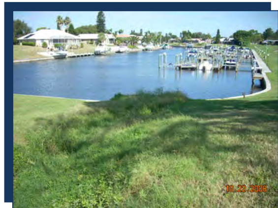
Photo: FC08 Outfall
