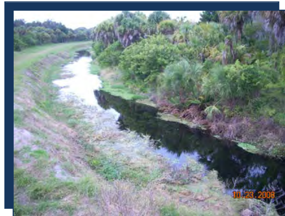
Photo: AC11 Downstream (Looking Southwest)
