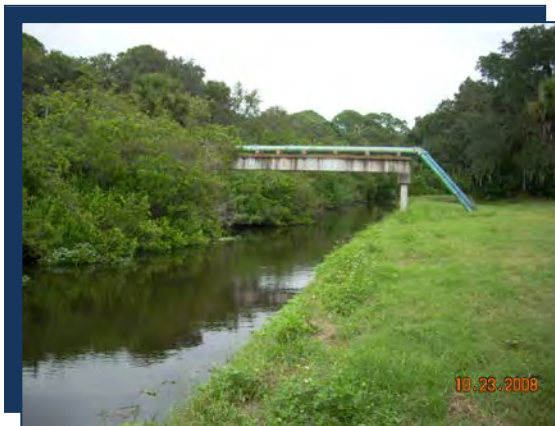
Photo: AC05 Upstream (Looking West)
