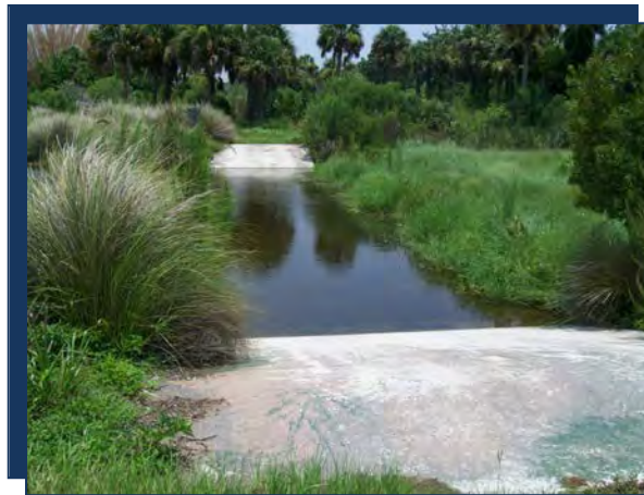
Photo: WM07 Preservation Area Weir
