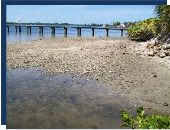
Photo: LBC1 Pier adjacent to outfall March 2009
