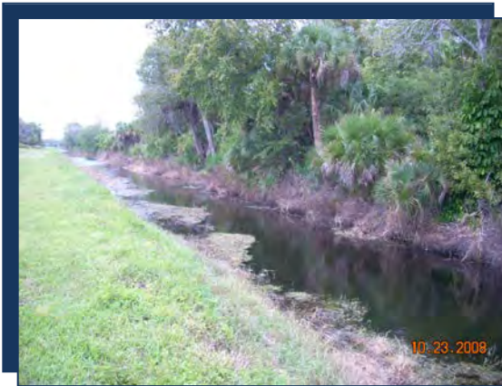
Photo: AC13 Downstream (Looking Southwest)
