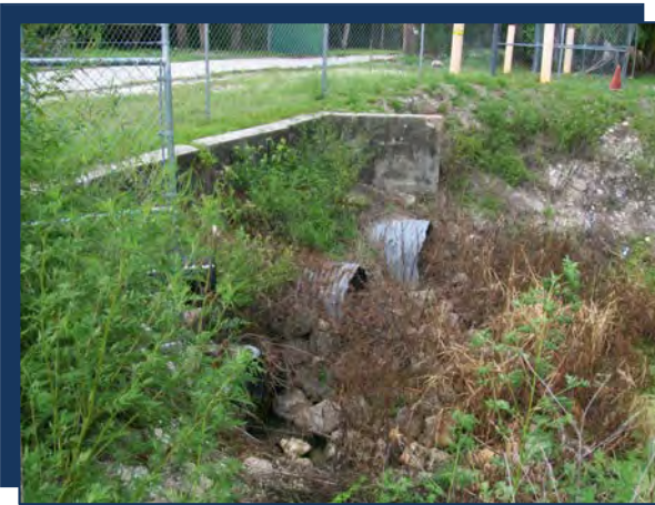
Photo: AC06 Culverts
