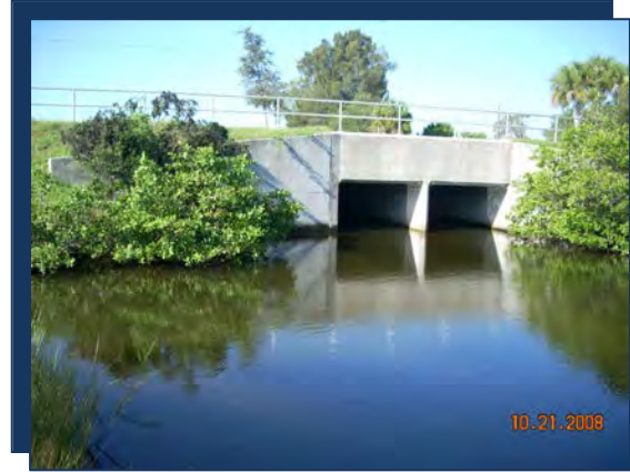
Photo: FC06 Downstream (Looking West)
