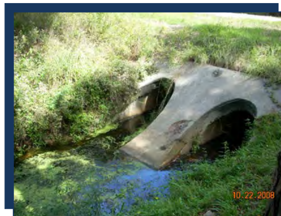
Photo: Woodmere Creek WM03-downstream culvert
