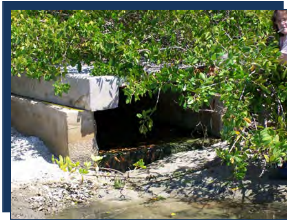
Photo: LBC1 Outfall (Looking North)
