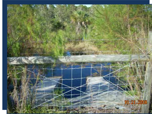
Photo: AN03 SW Treatment System
