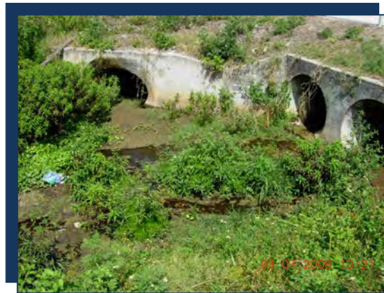
Photo: WM02 Downstream culverts (West of US41)
