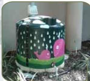
Cistern collecting rainwater for watering plants
