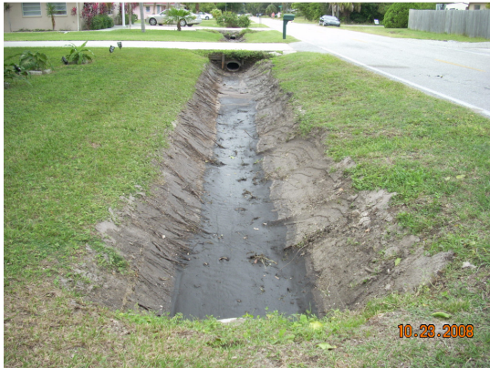
Photograph 3 Excavated Roadside Drainage Swale
