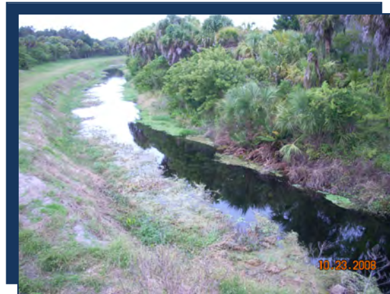
Photo: AC11 Downstream (Looking Southwest)
