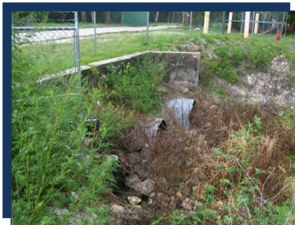
Photo: AC06 Culverts
