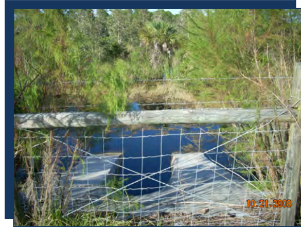
Photo: AN03 SW Treatment System
