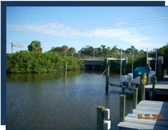
Photo: FC07 Upstream (Looking East)
