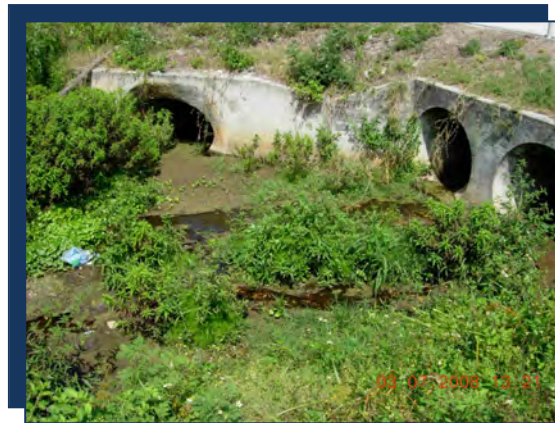
Photo: WM02 Downstream culverts (West of US41)
