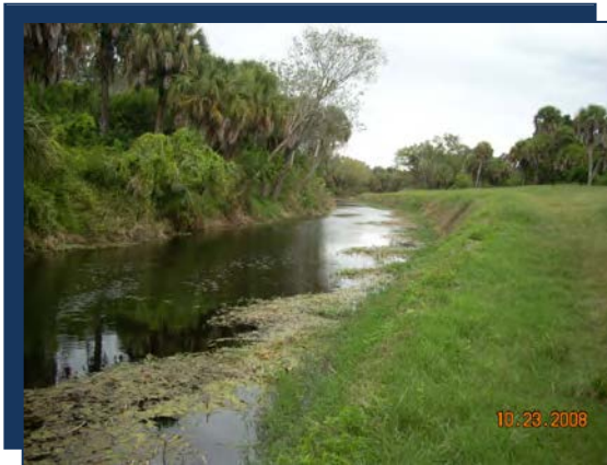
Photo: AC11 Upstream (Looking Northeast)
