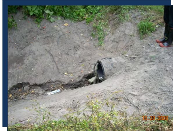
Photo: AC09 Culvert Outfall
