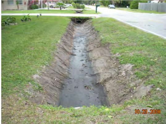
Photograph 3 Excavated Roadside Drainage Swale
