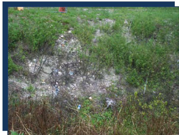
Photo: AC06 General Bank Condition
