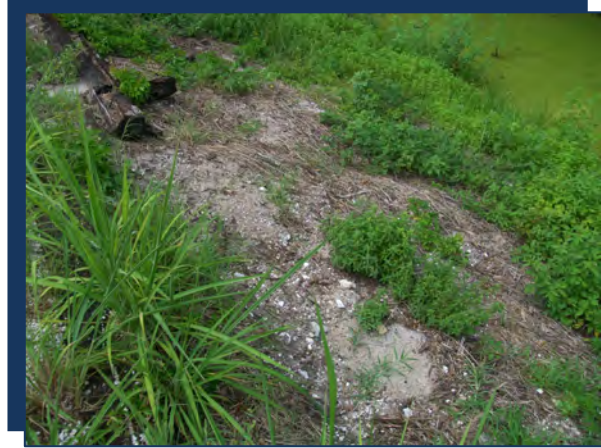
Photo: AC01: General Bank Condition
