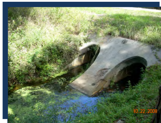
Photo: Woodmere Creek WM03-downstream culvert
