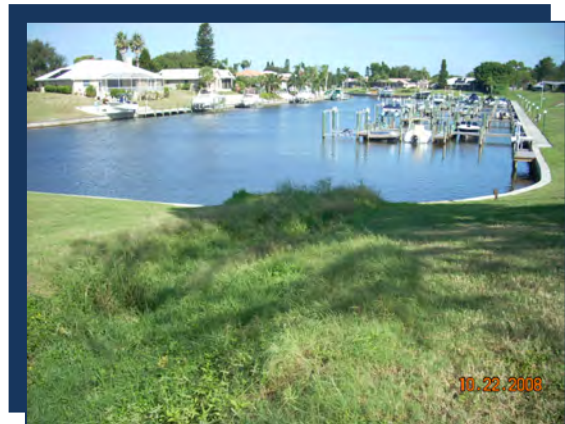
Photo: FC08 Outfall
