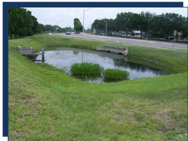
Photo: AC10 Adjacent Detention Pond
