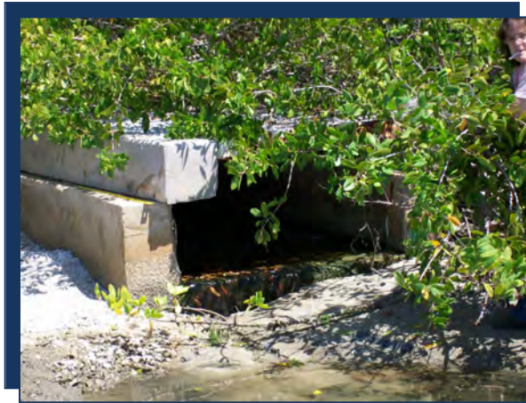
Photo: LBC1 Outfall (Looking North)
