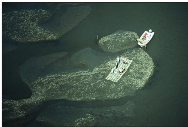
Figure 12. Aerial photograph of intertidal oyster reef construction in Inlet Creek, South Carolina, part of a six-year study by the Oyster Recovery Partnership (ORP). Photo courtesy of George Steele and Loren Coen, South Carolina Department of Natural Resources.
