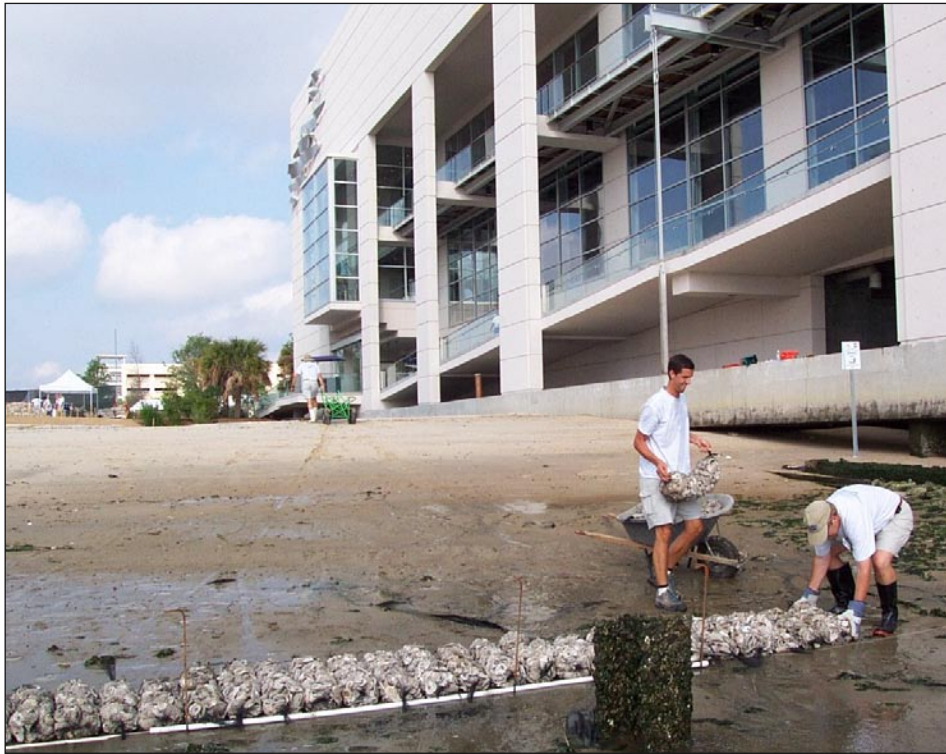
Figure 8. Volunteers use bags filled with recycled oyster shells to build large footprint reefs onto which oysters will settle, as part of South Carolina Oyster Restoration and Enhancement (SCORE) reef building project, South Carolina Aquarium. Photo courtesy of Loren Coen, Marine Resources Research Institute, South Carolina Department of Natural Resources.
