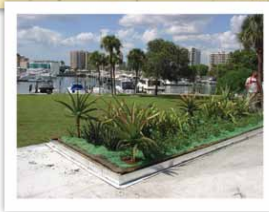
Green Roof at Island Park, Sarasota County.
